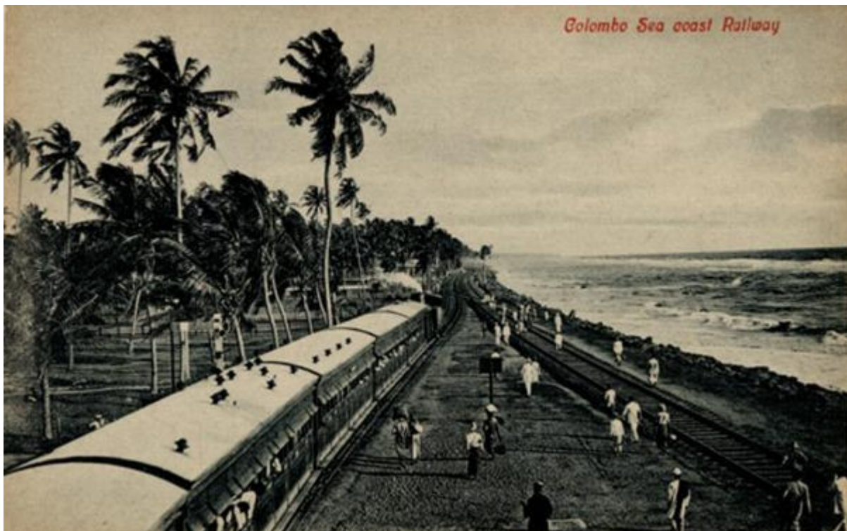
COAST LINE TRAIN (EARLY 20TH CENTURY) This is a scan of a postcard dating from the early 20th Century (although it must be later than 1912 because the line has been doubled). It shows a Coast Line suburban train with sun-shaded coaches headed by a CT class 4-4-0T tank engine and appears to be at taken at Bambalapitiya station but before coming of the proliferation of buildings on the land side.
