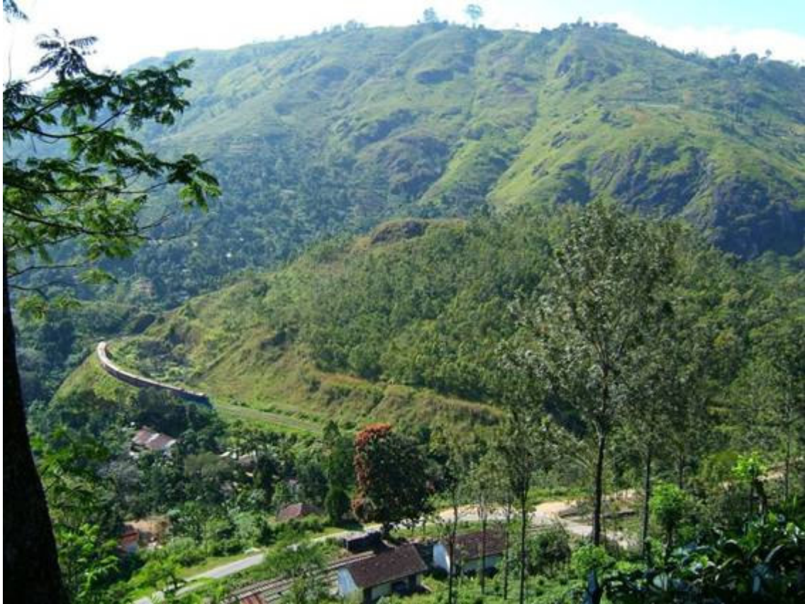
DEMODERA LOOP The only picture known to me of the complete Demodera Loop is that in plate 16 of my book. This picture is almost as complete, taken under much better conditions, and shows Podi Menike headed by an unidentified M6 locomotive travelling towards Badulla.
