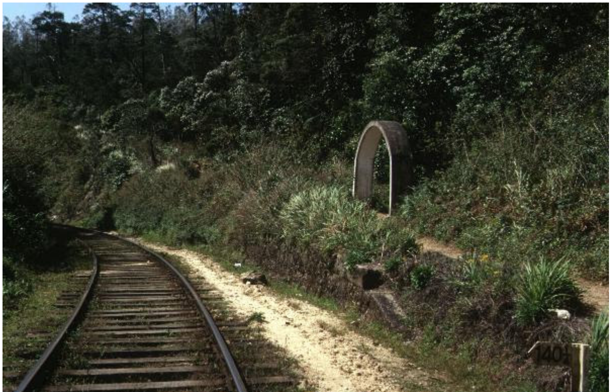
SUMMIT TEMPLE ENTRANCE As mentioned in RSL , two temples, one Buddhist and one Hindu, exist on the top of a cutting at the approach to the Summit Tunnel at Pattipola on the Main Line. One of the concrete arches used to reinforce the tunnel when it was repaired in 1981 was used as an entrance gateway to the path leading up to the temples.
