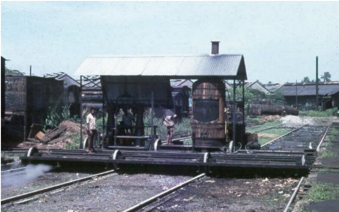
DUAL GAUGE TRAVERSER AT DEMATAGODA This links the roads in Shop 26 with a number of sidings both broad and narrow gauge and, although now operated electrically (below), was steam operated until about 1983 (above). Although at Dematagoda, Shop 26 is an outpost of the CME Department at Ratmalana.
