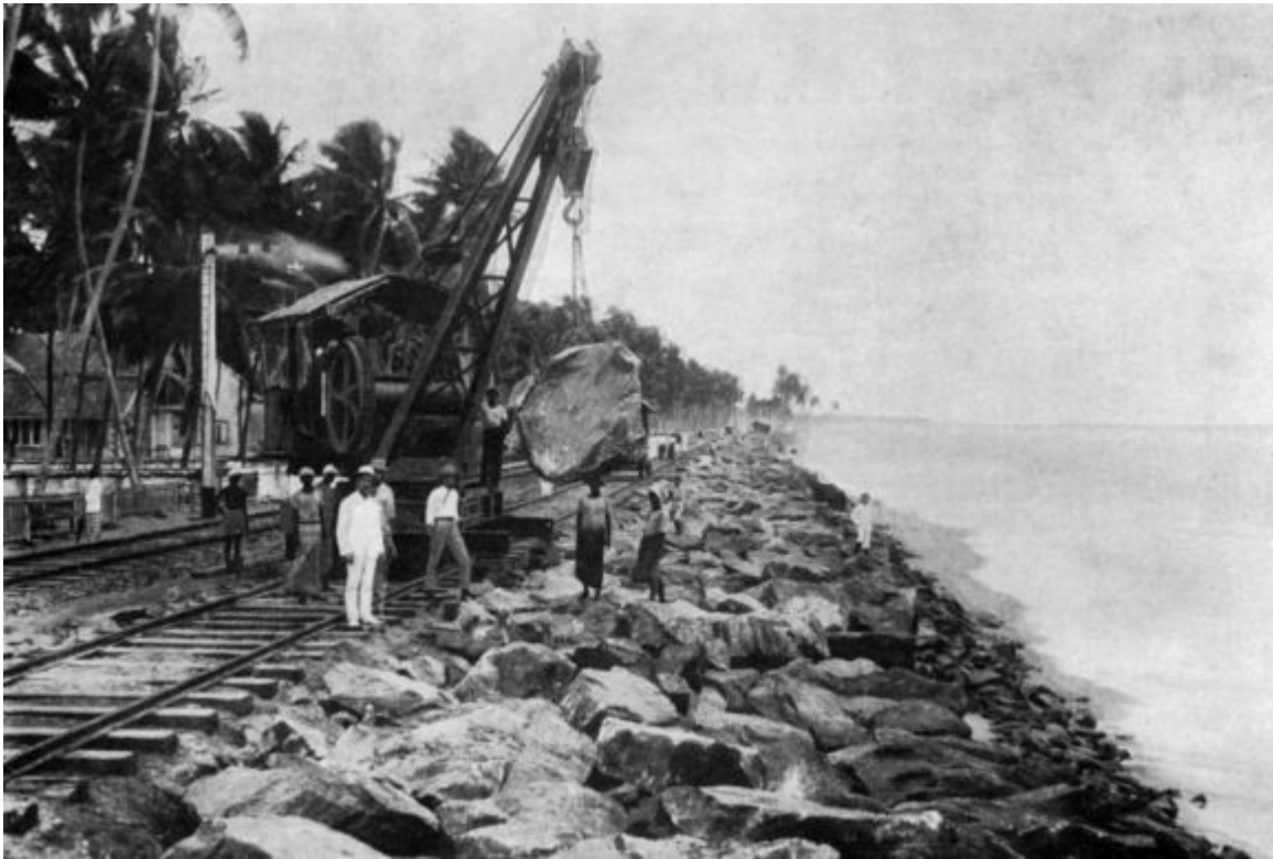
LARGE STONE PLUMBS TO STABILISE THE COAST LINE Erosion of the Coast Line has always been a serious problem and large stone plumbs were brought from a quarry at Ragama to stabilise the line. [Administration Reports, 1911]
